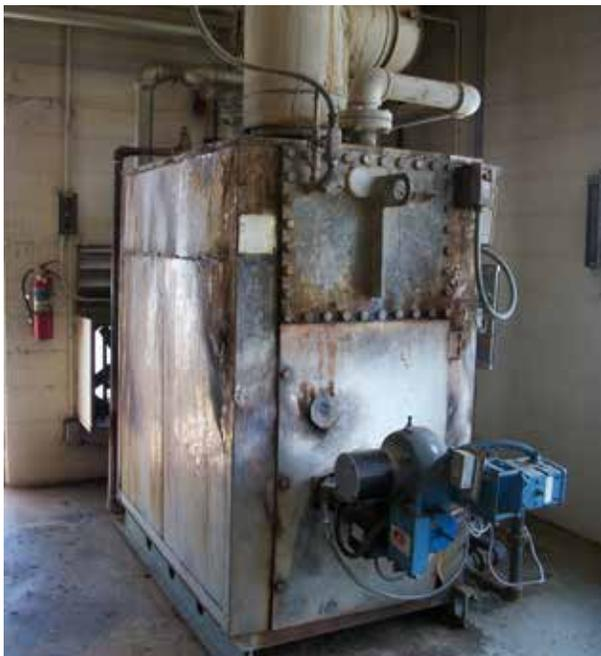
The rate study will help the District make sure the District’s Sewer Service Charges fully funds operations and maintenance activities as well as the replacement of critical operational equipment like this Digester Boiler unit which is used to keep the Biosolids Digester at optimal temperatures.
