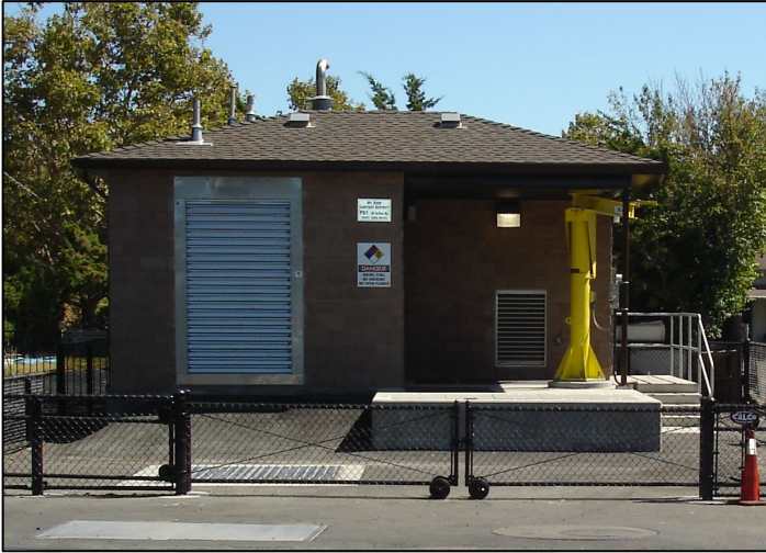
Pump Station No. 1
