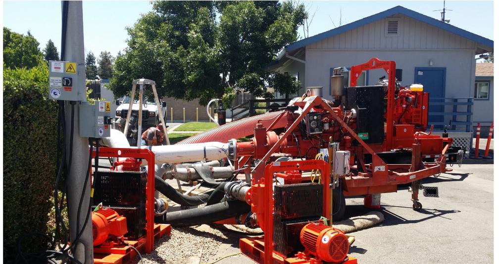
To allow construction in the pump station wet well, 100% of incoming flow must be temporarily pumped around the influent pump station and into the treatment plant for processing.
