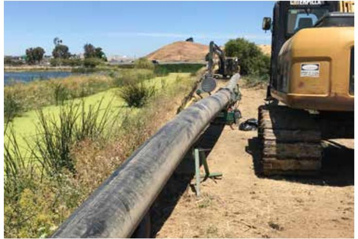
The contractor here is fusing HDPE bypass pipe for Peyton Slough.
