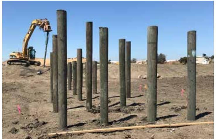
Installing piles in pond A2 - These piles will support the boardwalk and viewing platform.
